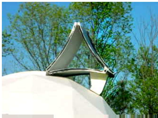
Since the door must be a bit longer than 8' (the length of the masonite board), to "stretch" the door, I used a couple of pieces of aluminum extrusion to sandwich the door at each end as shown in the figure.
